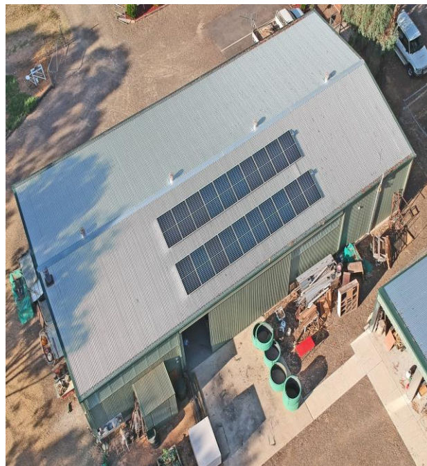
Aerial view of the solar panels
