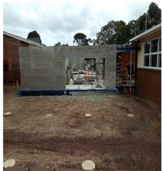
Rear view. The gap between the camera and the block wall will be filled by a very large timber deck; doors will fill the gap in the wall.
