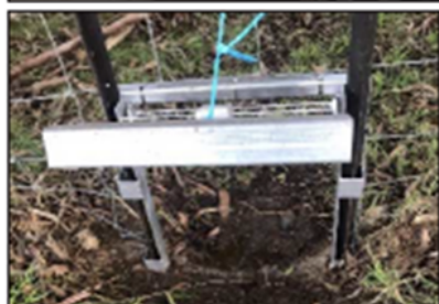
Above: Wombat swing gates are easy to install and should be placed on well-used wombat tracks. Installation is simple and instructions are provided. Once installed, it is best to tie the gate up for a couple of weeks so the wombats slowly get used to the change in the fence. The gate is then lowered.
